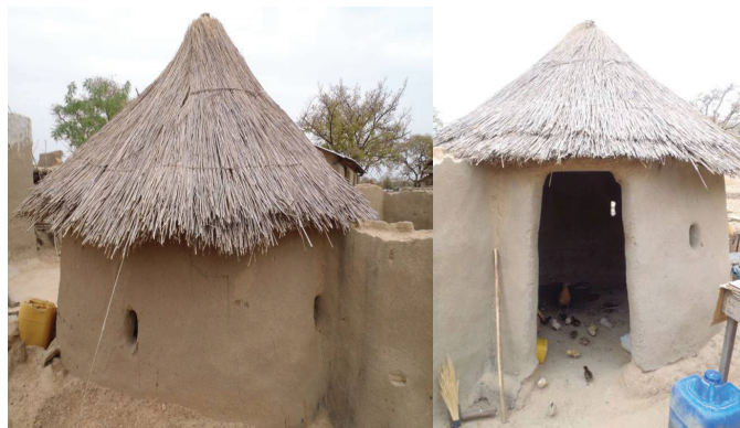
Figure 11. Mud housing with thatch roof
